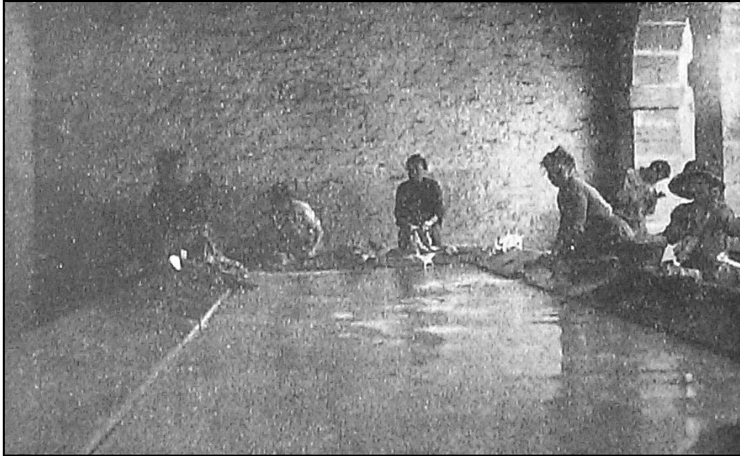
Public Washing Place – France, Chalindry
